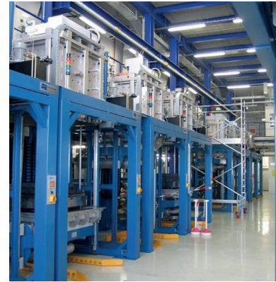
Fig. 9 Several equally sized batch furnaces, forming a "quasi-continuous" sintering technology network
